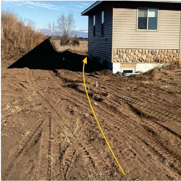
Gas meter location flagged left side of house
