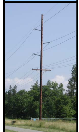
Typical 115 kV Transmission Structure With Distribution Underbuild
